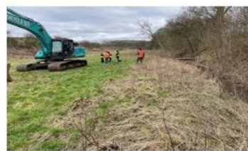
Site before works with old channel to right Credit: EA
