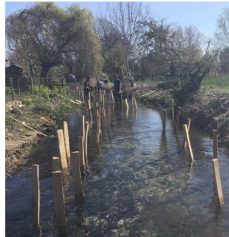
Berm installation
